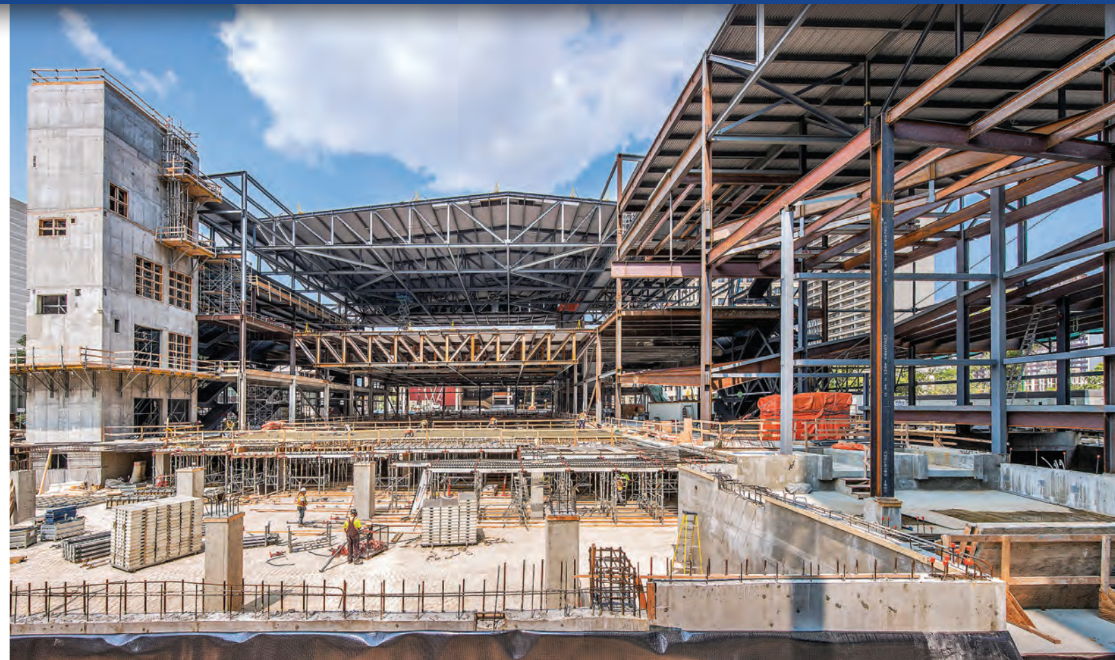
Structural steel framing for the expansion
