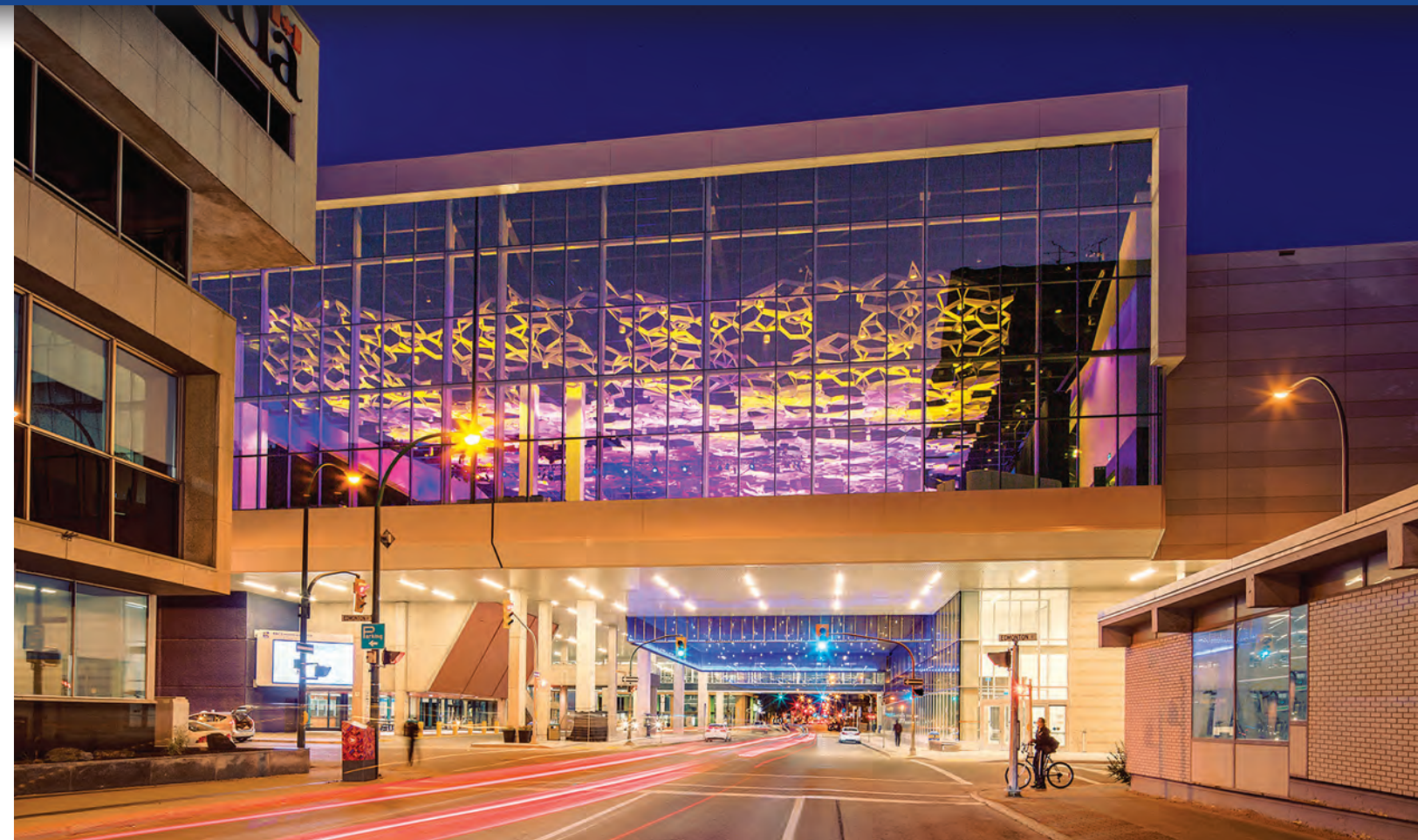
View of City View Room from York Avenue
